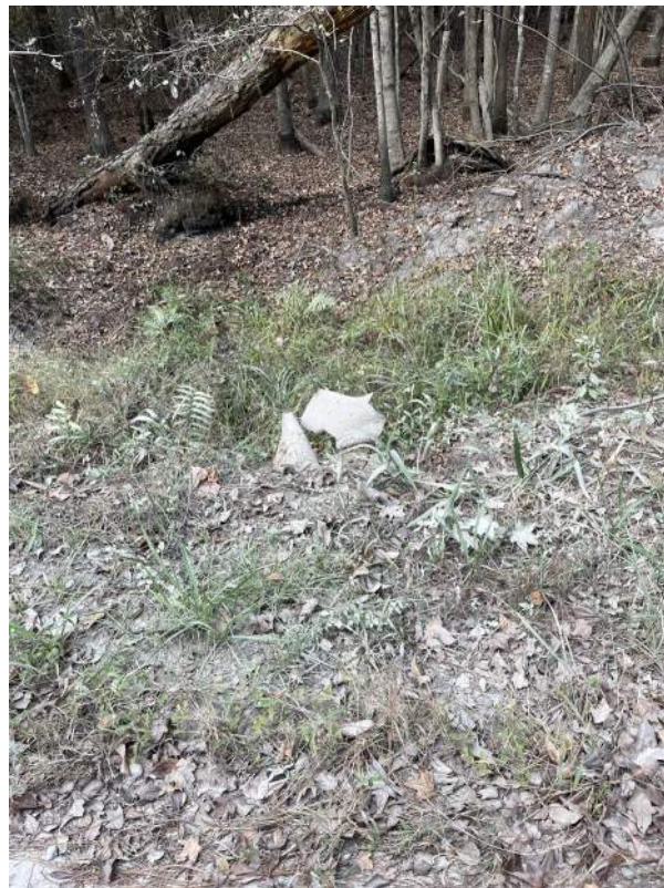
Figure 37: Downstream of Osteen Road near Crossing #3. The view is facing downstream.
