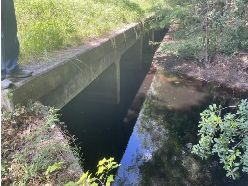
Figure 13: Crossing #2 along US Highway 80 that consists of (6) 9'x5' box culverts. The view is facing upstream.
