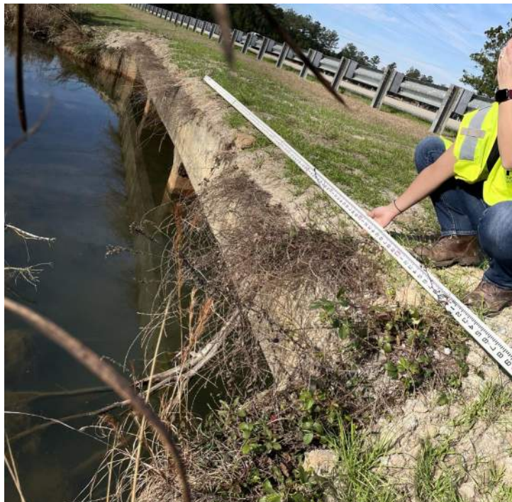
Figure 52: Crossing #2 along Highgate Boulevard consisting of a 12'x4' triple box culvert. The level rod is resting horizontal to the sides of one of the culvert's openings. The view is facing upstream.
