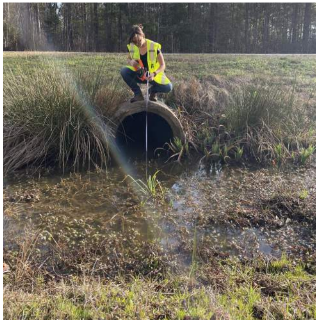
Figure 58: Crossing #6 along Little Neck Road consisting of a 30" RCP. The tape is resting on the invert of the culvert. The view is facing downstream.
