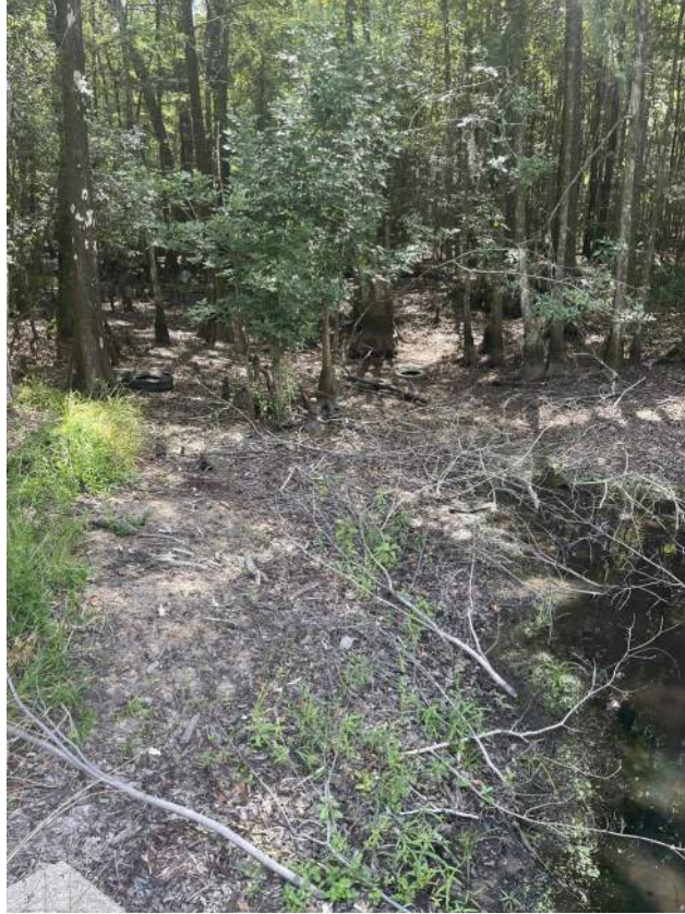
Figure 27: The conveyance system downstream of Meldrim Road near one of the Crossing #7 box culverts. The view is facing downstream.
