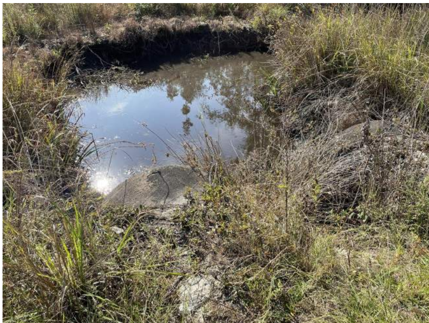
Figure 5: Crossing #3 along Blue Jay Road that consists of (2) 36" RCPs. The view is facing downstream.
