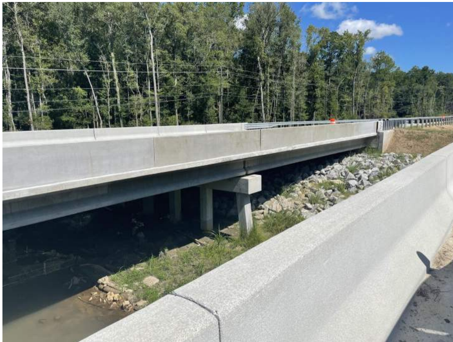
Figure 41: Crossing #5 along Jimmy Deloach Parkway which consists of a bridge. The view is facing upstream.
