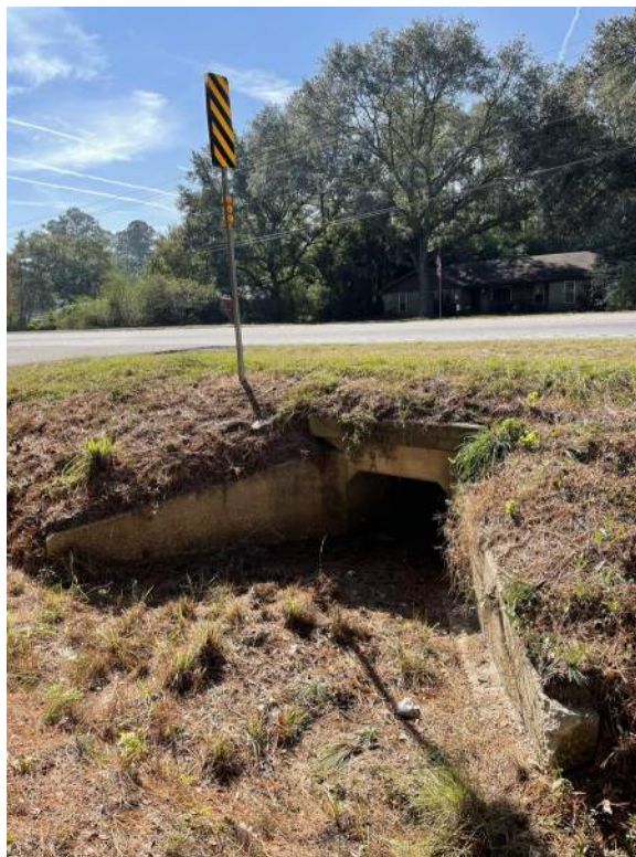
Figure 19: Crossing #5 along US Highway 80 that consists of a 5'x4' box culvert. The view is facing downstream.
