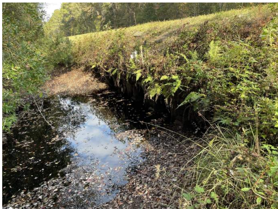
Figure 1: Crossing #1 along Midland Road that consists of (7) 36" RCPs. The upstream inverts are approximately half-way full of water. The view is facing downstream.
