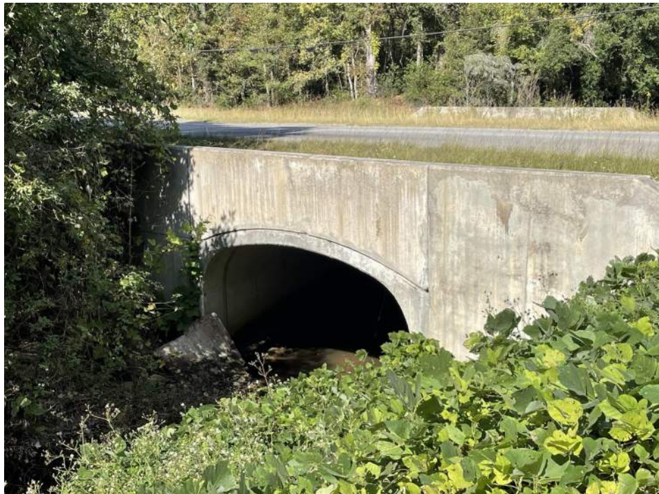
Figure 64: Crossing #3 along Little Neck Road which consist of a 12'x8' Con/Span. The view is facing downstream.
