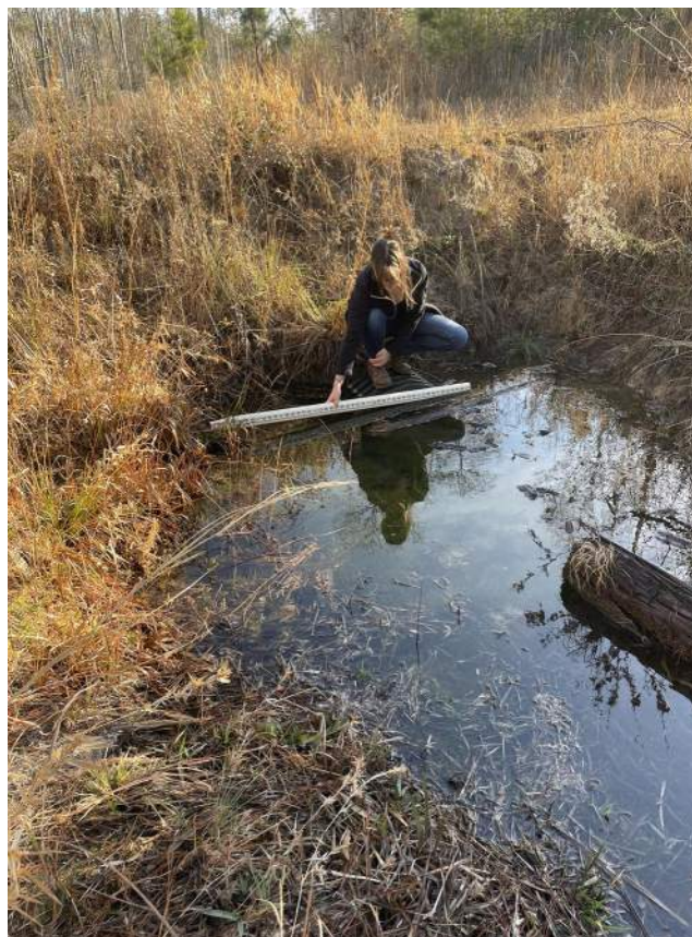
Figure 31: Crossing #1 along Osteen Road. The level rod is rested horizontal to the sides of the 30" CPP. View is facing upstream.
