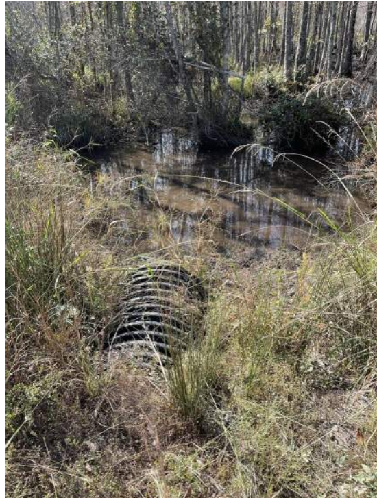
Figure 46: Crossing #3 along Orendorff Road that consists of (7) 24" CPP. The view is facing downstream.
