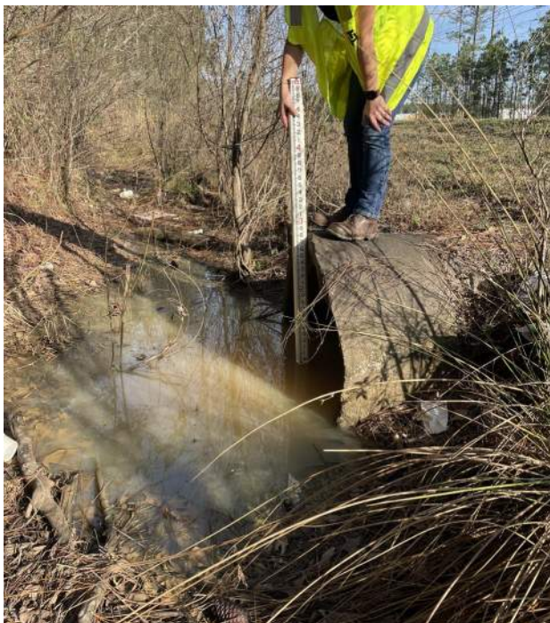
Figure 59: Crossing #7 along Little Neck Road consisting of a 36" RCP. The level rod is resting on the invert of the culvert. The view is facing downstream.
