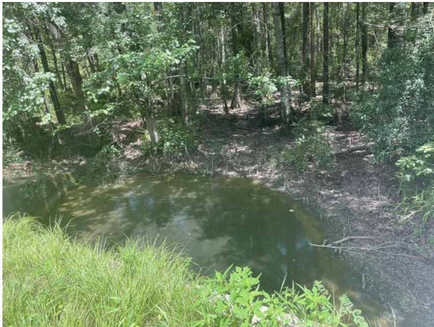
Figure 14: Upstream conveyance system of US Highway 80 (near triple box culvert). The view is facing upstream.
