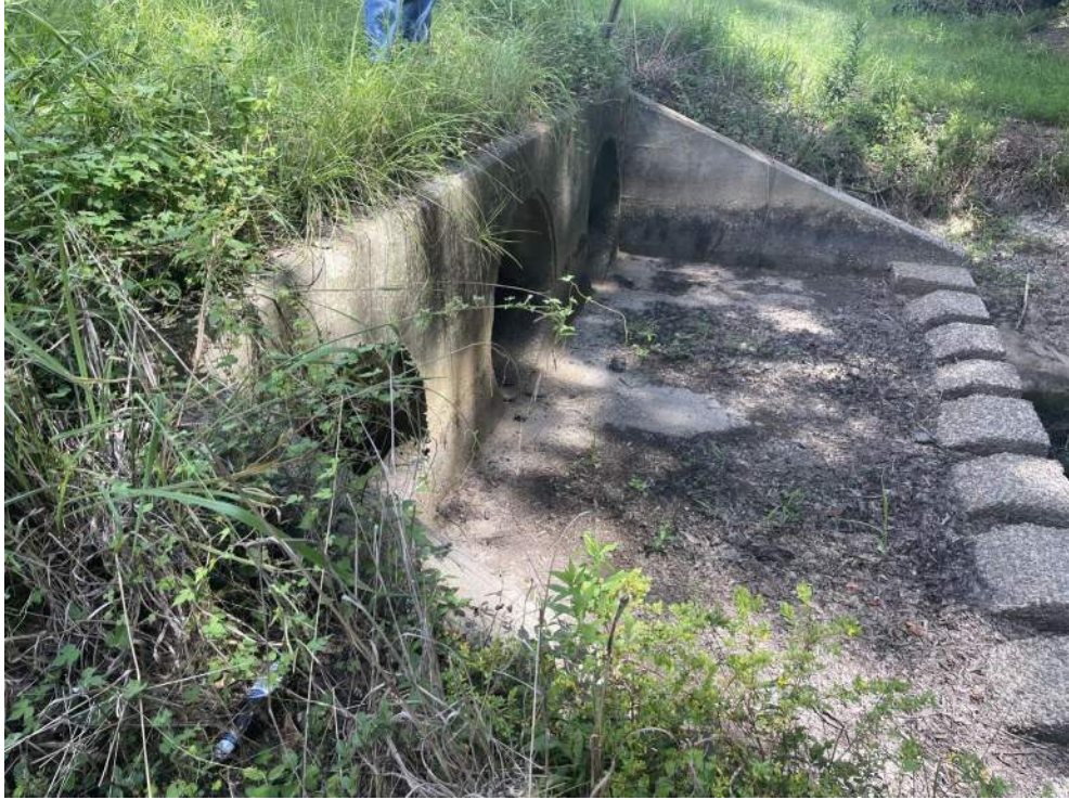
Figure 23: Crossing #7 along Meldrim Road that consists of the second set of (3) 42" RCPs. The view is facing upstream.
