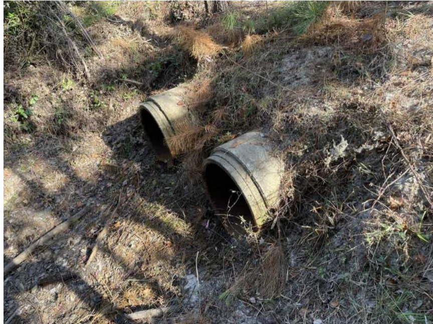
Figure 29: Crossing #8 along Meldrim Road that consists of (2) 24" RCPs. The view is facing downstream.
