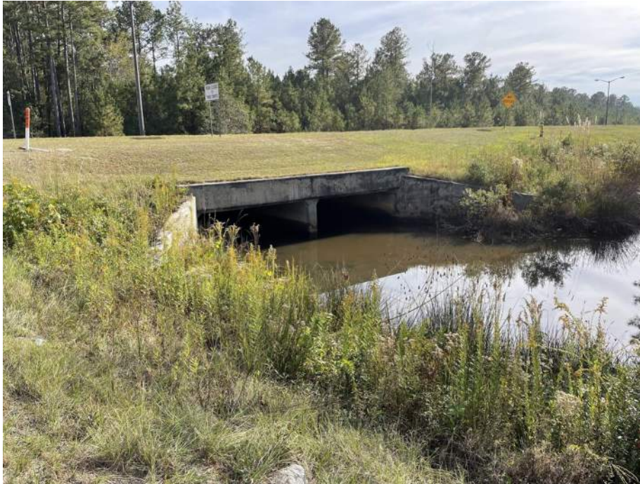
Figure 57: Crossing #5 along New Hampstead Parkway consisting of a 12'x5' double box culvert. The view is facing downstream.
