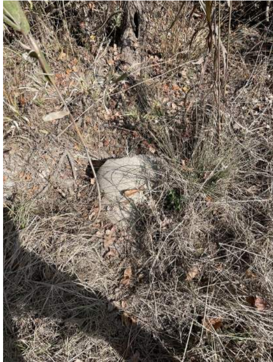
Figure 34: Crossing #2 along Osteen Road that consists of an 18" RCP. View is facing upstream.
