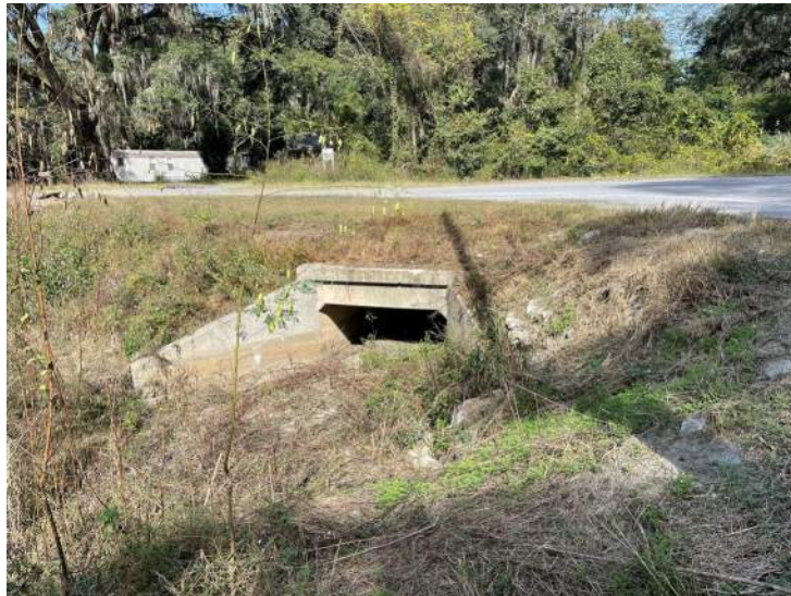
Figure 61: Crossing #1 along Little Neck Road consisting of an 8'x4' box culvert. The view is facing downstream.
