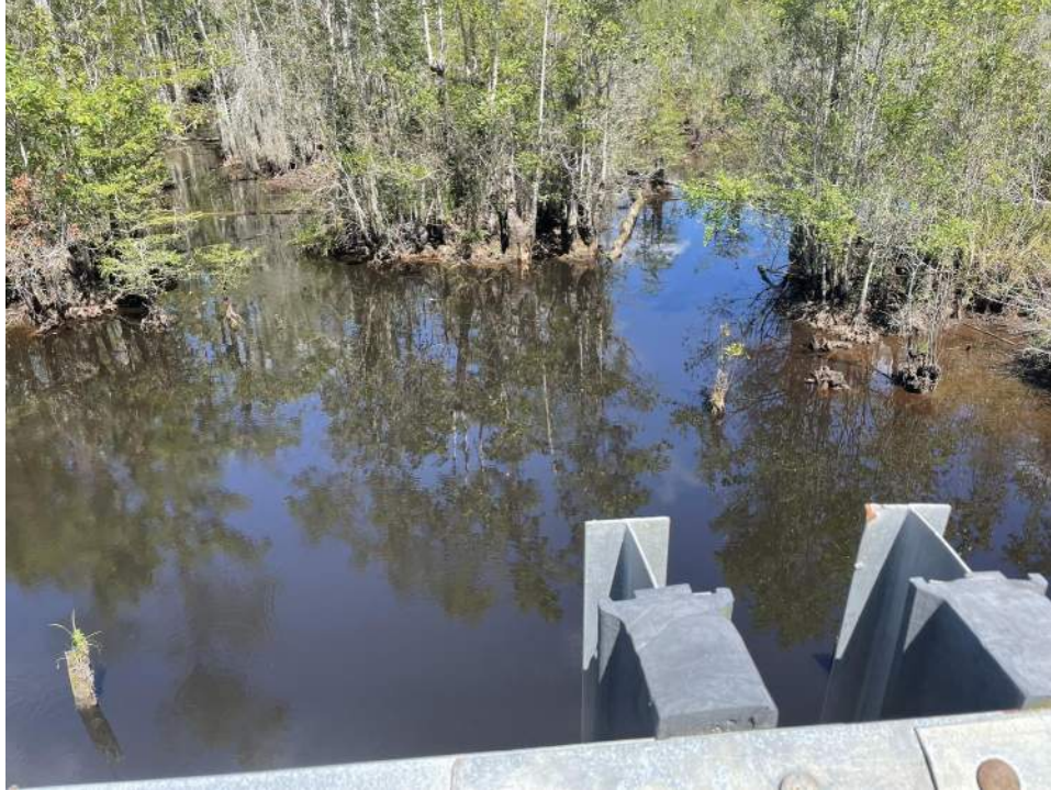
Figure 40: Downstream channel of the Little Ogeechee River that passes under Osteen Road at Crossing #4. The view is facing downstream.
