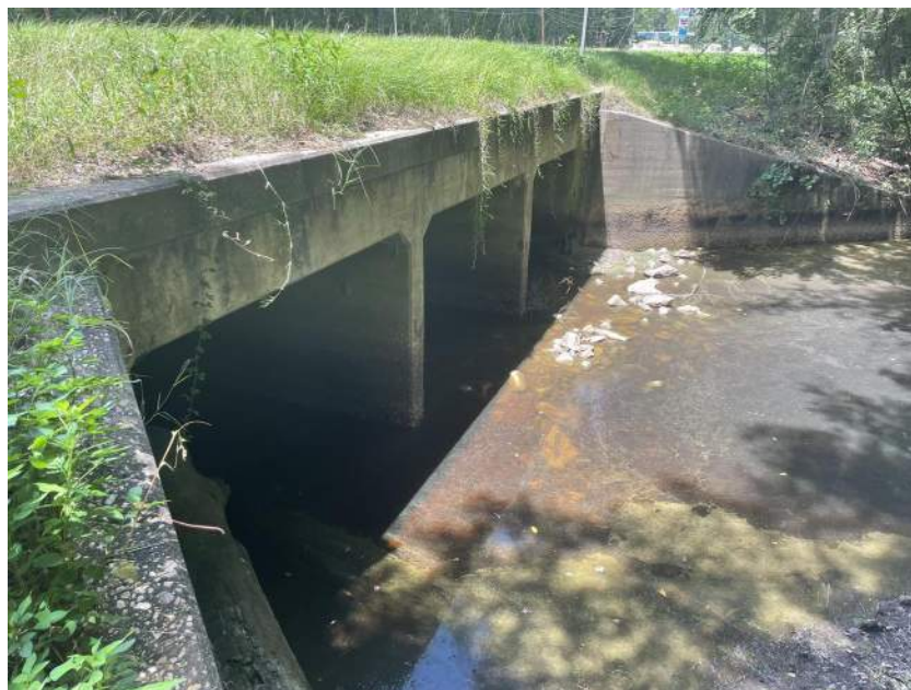
Figure 12: Crossing #2 along US Highway 80 that consists of a 9'x5' triple box culvert. The view is facing downstream.
