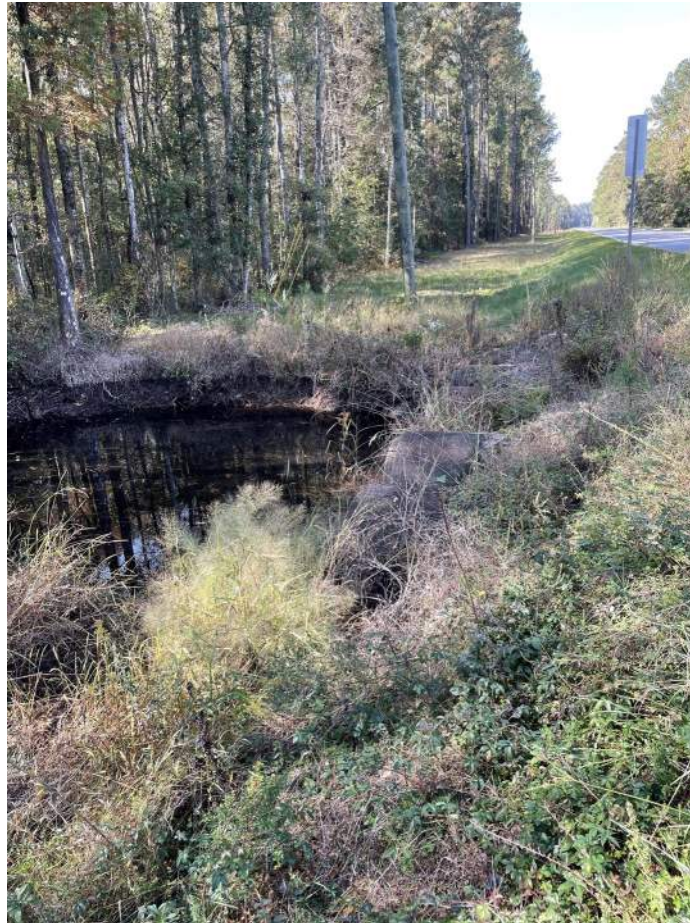
Figure 7: Crossing #4 along Blue Jay Road that consists of (4) 42" RCPs. The view is facing west on the downstream side of Blue Jay Road.
