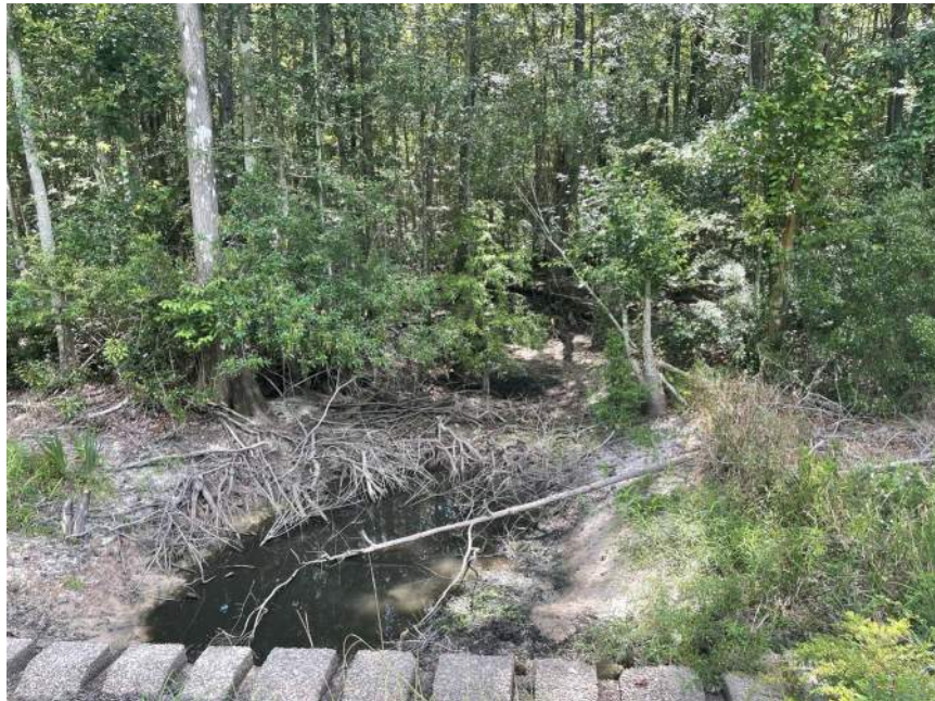
Figure 28: The conveyance system downstream of Meldrim Road near one set of the Crossing #7 RCPs. The view is facing downstream.
