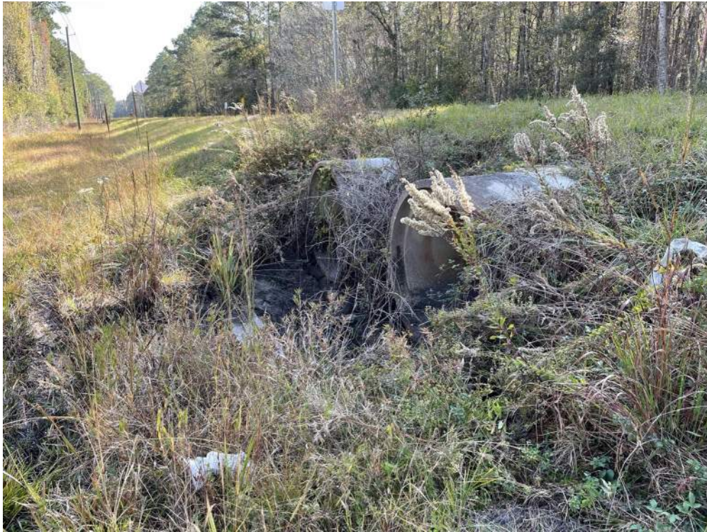
Figure 10: Crossing #5 along Blue Jay Road that consists of (2) 42" RCPs. The view is facing downstream.
