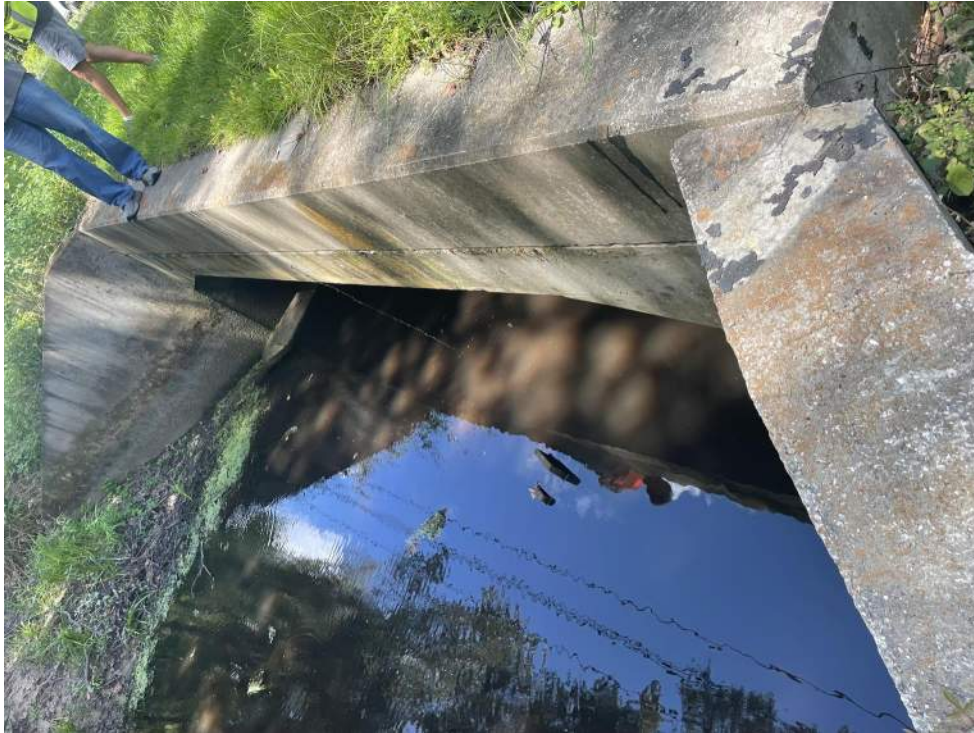
Figure 25: Crossing #7 along Meldrim Road that consists of the second 20'x3' box culvert. The view is facing upstream.
