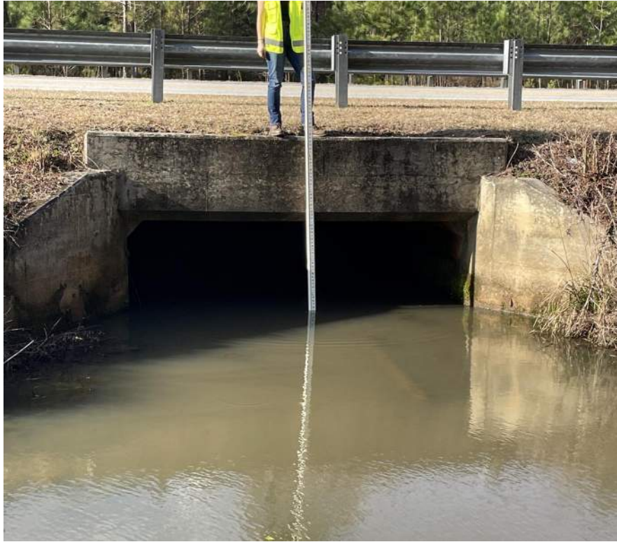
Figure 55: Crossing #4 along Highgate Boulevard consisting of a 10'x4' box culvert. The level rod is resting on the invert of the culvert. The view is facing downstream.
