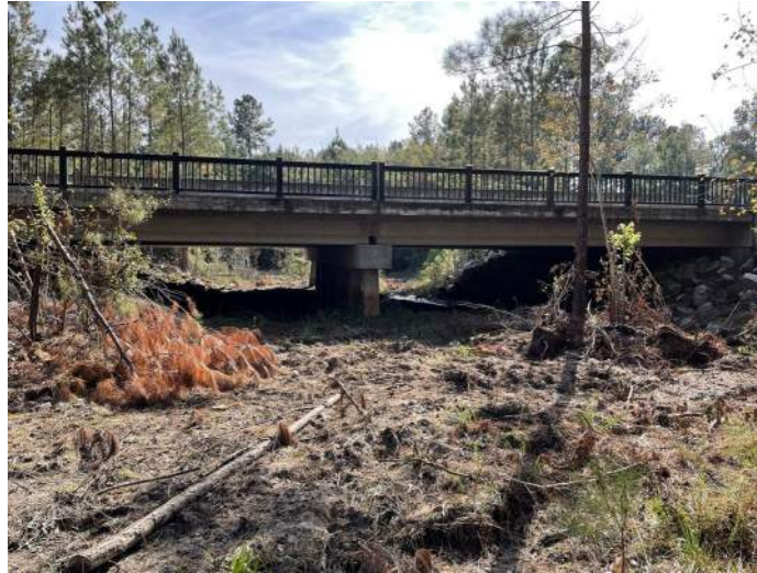
Figure 49: Crossing #1 along Highgate Boulevard which consist of a bridge. The view is facing upstream.
