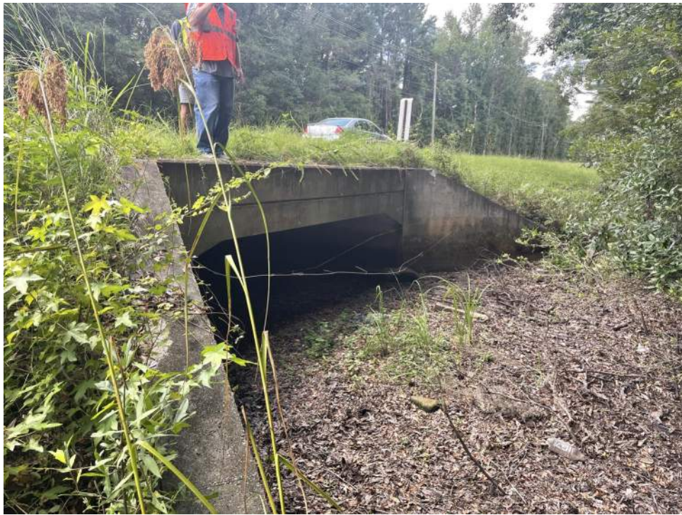
Figure 24: Crossing #7 along Meldrim Road that consists of the first 20'x3' box culvert. The view is facing upstream.
