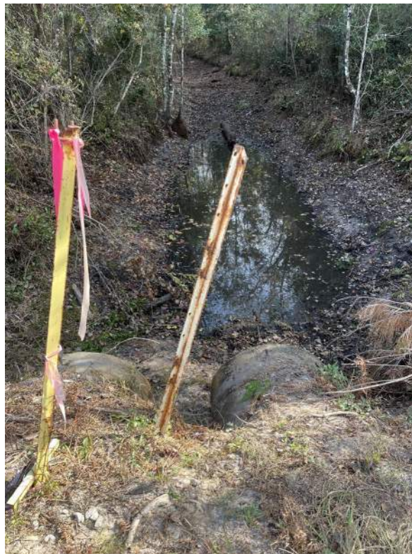
Figure 30: Channel downstream of Meldrim Road, near Crossing #8. The view is facing downstream.
