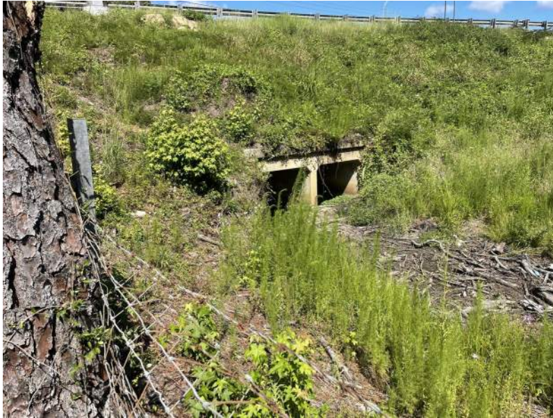
Figure 48: Crossing #4 along Little Neck Road that consists of a 6'x6' double box culvert. The view is facing upstream.
