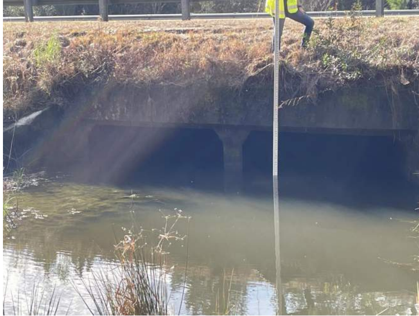
Figure 53: Crossing #3 along Highgate Boulevard consisting of a 7'x4' double box culvert. The level rod is resting on the invert of the culvert. The view is facing downstream.
