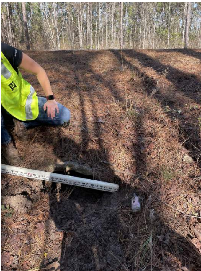
Figure 43: Crossing #1 along John Carter Road. The level rod is rested horizontal to the sides of the 24" RCP. The view is facing downstream.
