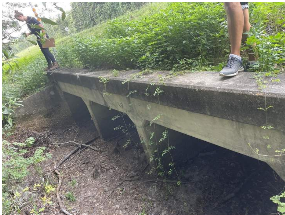
Figure 17: Crossing #3 along US Highway 80 that consists of a 6'x4' triple box culvert. The view is facing downstream.
